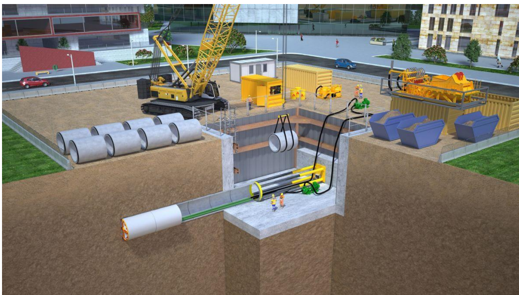
Figure 47: Microtunnelier
